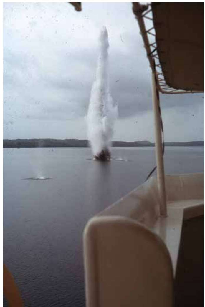
Above, blowing a hole in the reef at Yap Harbor to create a buoy.
